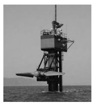
**Figure 13.6** SeaFlow with its rotors raised (Source: http://en.wikipedia.org/wiki/Marine\_Current\_Turbines)
