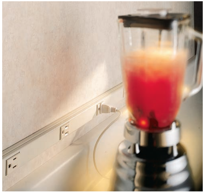
Figure 18-18 A multioutlet assembly installed above the backsplash of a kitchen countertop. Courtesy of The Wiremold Company, West Hartford, CT 06110.
