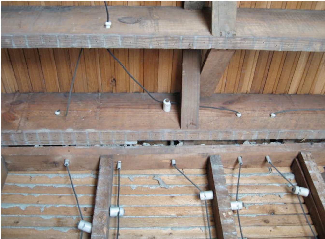
Figure 4-5 Photograph of a typical knob-and-tube wiring from the 1930s.
