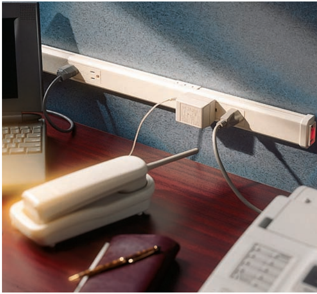
Figure 18-15 A typical metal multioutlet assembly. Multioutlet assemblies are permitted to be run through (not within) a dry partition when no outlets are located within the partition, and all exposed portions of the assembly can have the cover removed. Nonmetallic multioutlet assemblies are also available. Courtesy of The Wiremold Company, West Hartford, CT 06110.
